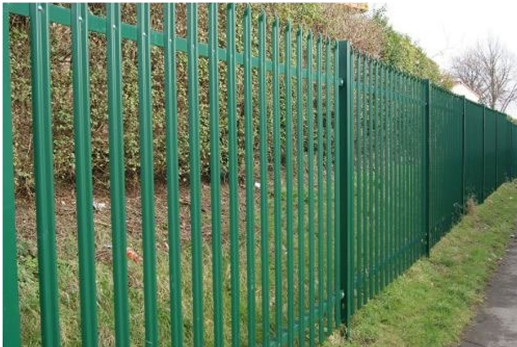
Plate 4.14 Typical Palisade Fencing
