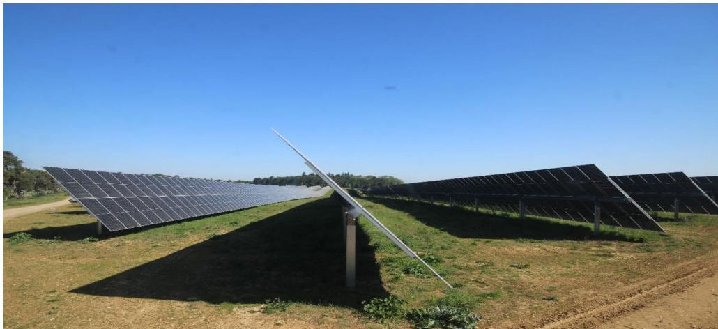
Plate 4.1 Typical Tracking Panels
