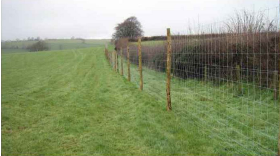
Plate 4.13 Typical Wire Mesh Fencing
